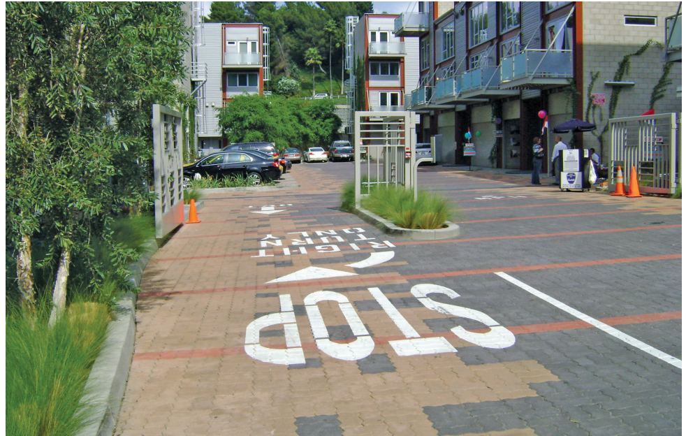
Shown: Serpentine 80mm in solid Charcoal, Red and Cream installed in a basketweave pattern.
